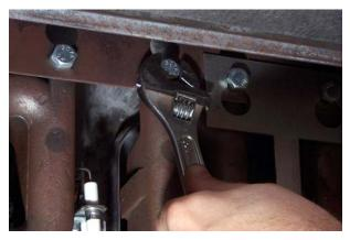
Loosening burner bolts prior to burner removal.
